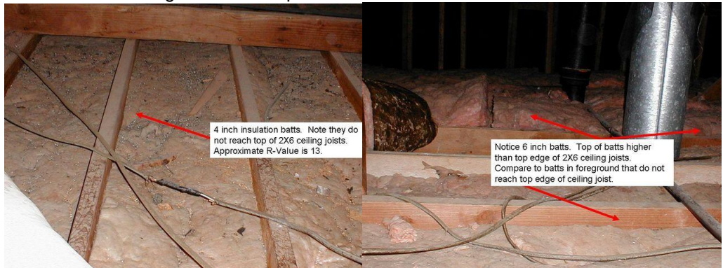
Above two pictures show 4 in. batts and thicker over-layment of 6 in. batts
